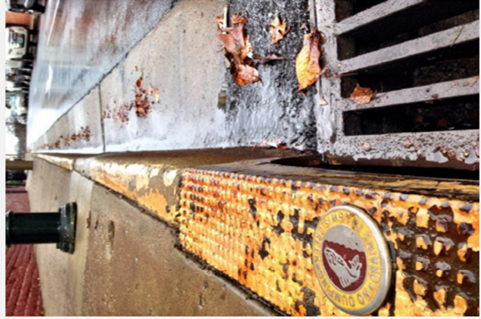
Storm drain in downtown Staunton
