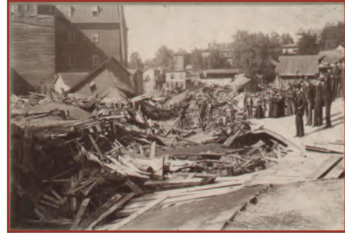
Damages From 1896 Flood Source: City of Staunton—Local Citizen
